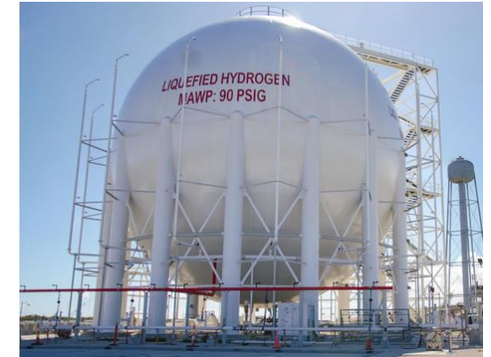
NASA Artemis programme: World's largest LH2 tank (1.25 M gal = 4.730 m 3 ) https://twitter.com/NASAGroundSys/status/1645510449071357959
